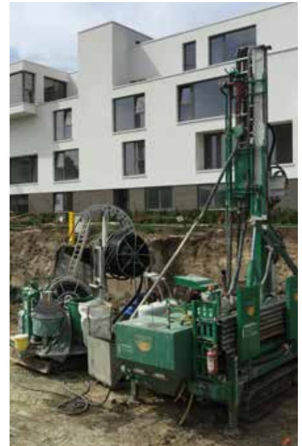
Drilling for ground source heat pumps
